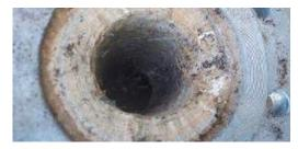
Struvite scale was building up in the centrate line from the centrifuge, causing flow restrictions and increasing the need for manual maintenance and pipe bypassing.
