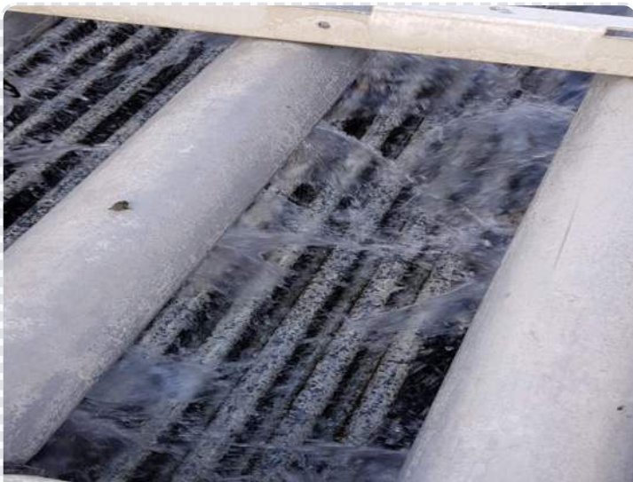
Heavy scale on cooling surfaces
