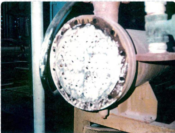
Heat exchanger tubes blocked by scale
