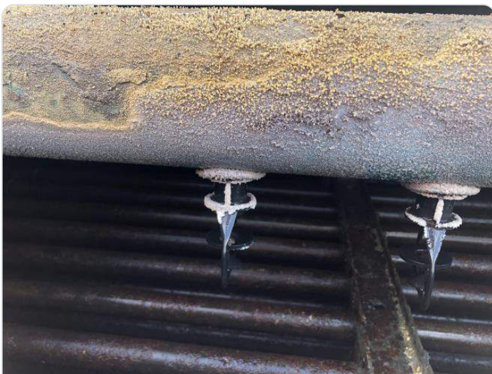
Scaling on nozzles before trial
