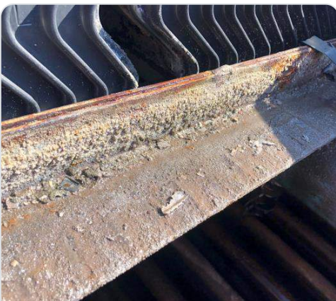
Condenser 4 tubes largely scale free
