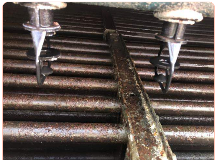
Clean nozzles after 3 months operation
