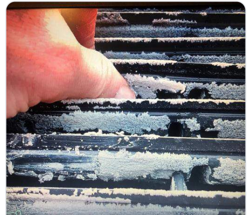
Scale on eliminators before treatment
