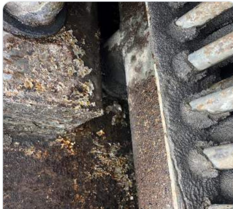
Condenser 3 tubes and frame with scale
