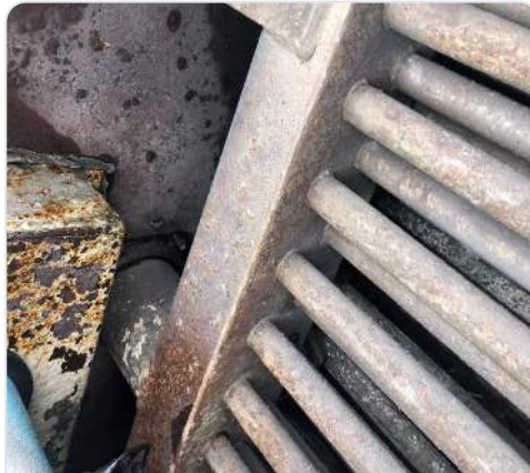
Condenser 3 tubes and frame with scale
