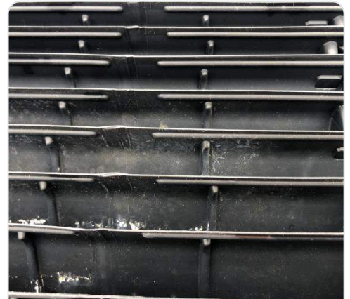
Scale on eliminators before treatment
