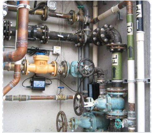
Water feature filtration system
