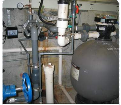
Water feature filtration system
