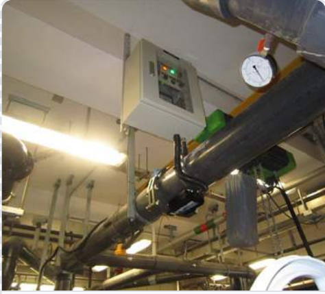
Water feature pipework and controls
