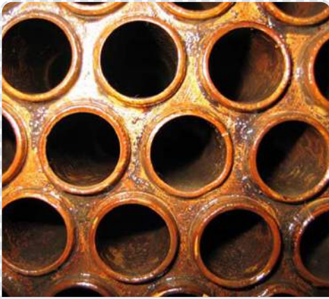
Clean condenser tube surface after biofilm removal
