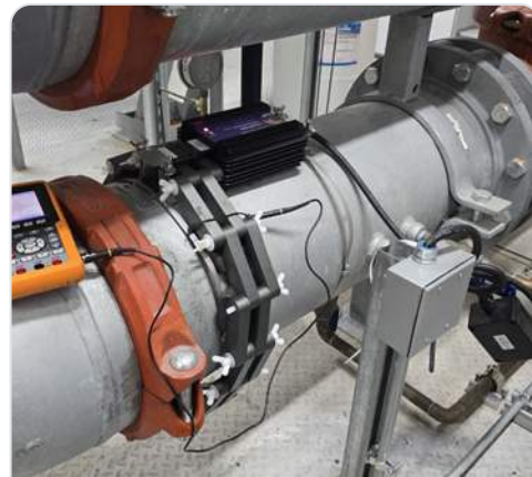
Additional HydroFLOW® i14 units on remaining loops
