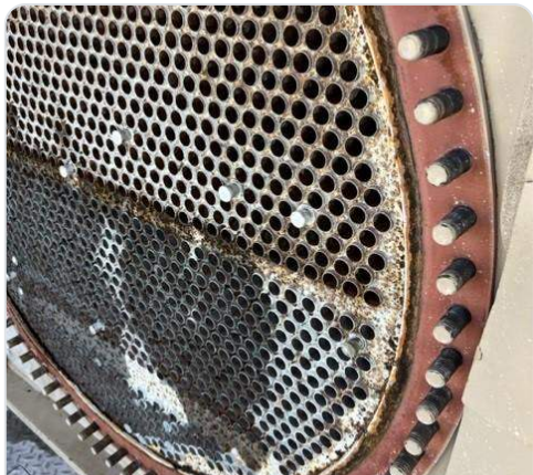
Tube sheet showing scale deposits before treatment
