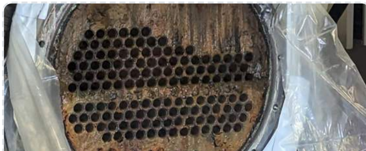
Tube sheet showing minimal soft scale
