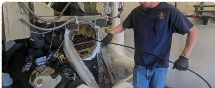
Chiller inspection showing minimal soft scale
