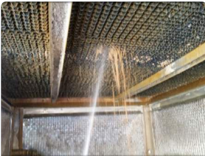
Manual hose cleaning of fouled tower
