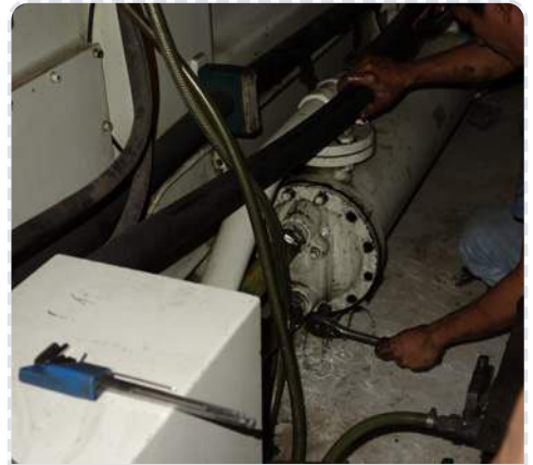
Machine maintenance due to overheating and scaling
