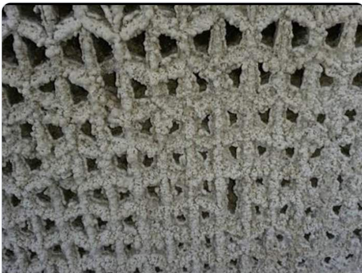
Heavy scale on drift eliminators
