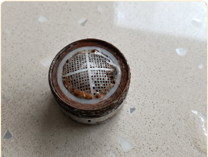
AFTER Jet breaker cleared of biofilm
