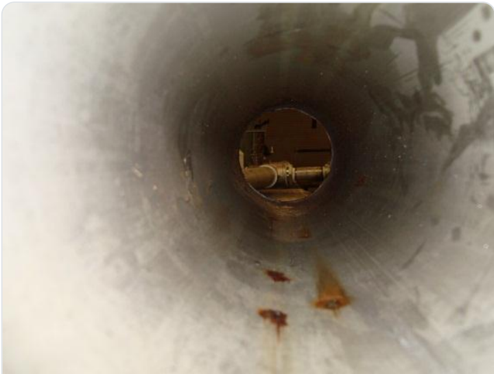
Contaminated pipe spool section
