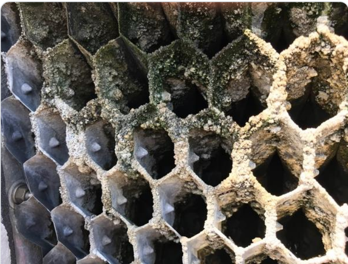
Heavy scale and biofilm on cooling-tower
