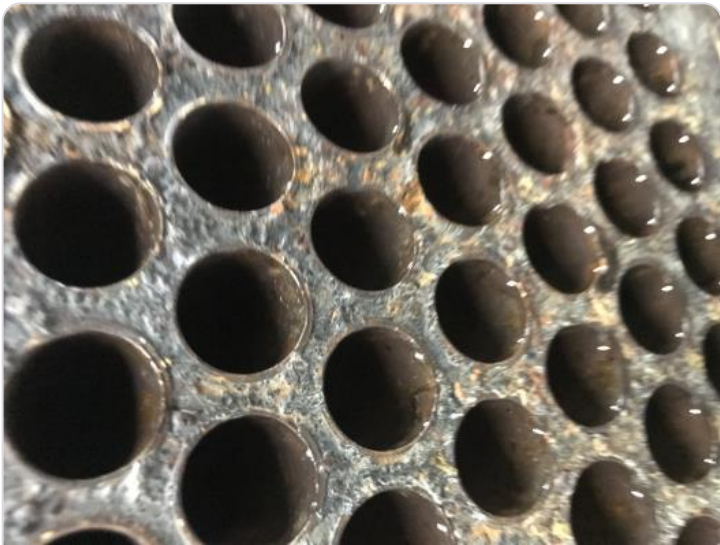
Cleaner chiller tubes after treatment
